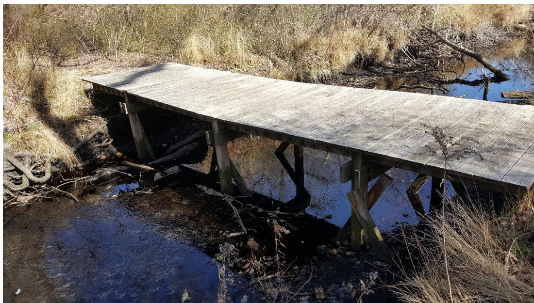
Figure 8: Bridge over central ditch.
