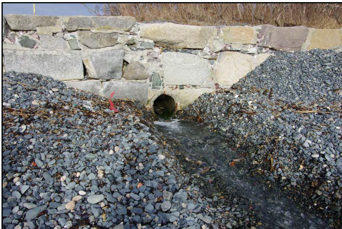
Photo 2: Existing seawater effluent pipe at seawall.
