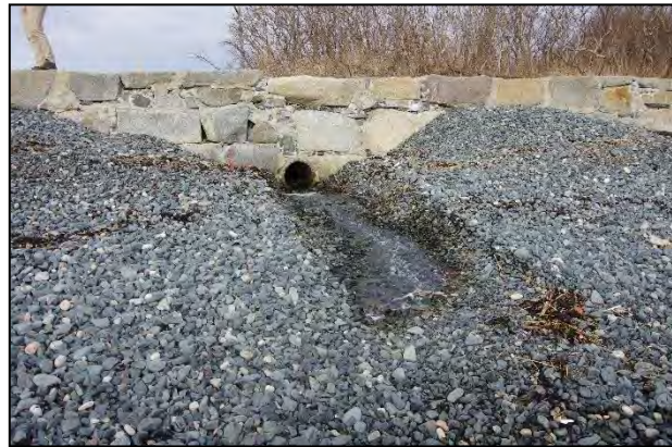
Existing 15" Discharge Pipe at Seawall
