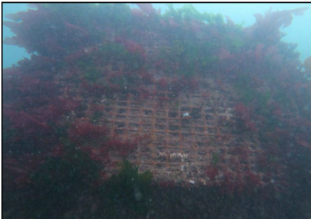
Photo 6: View of intake box screen
